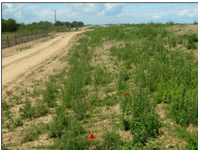
A229 roadworks, habitat. Photo by Geoffrey Kitchener, June 2011
