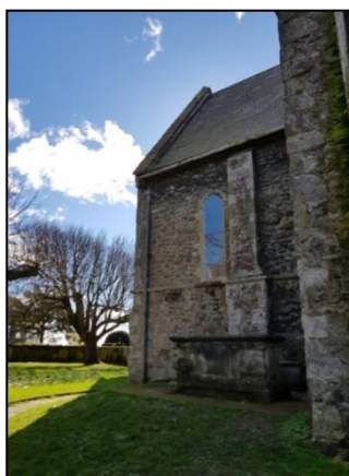
Church roof, Folkestone. Photos by Sue Buckingham, 1 March 2019
