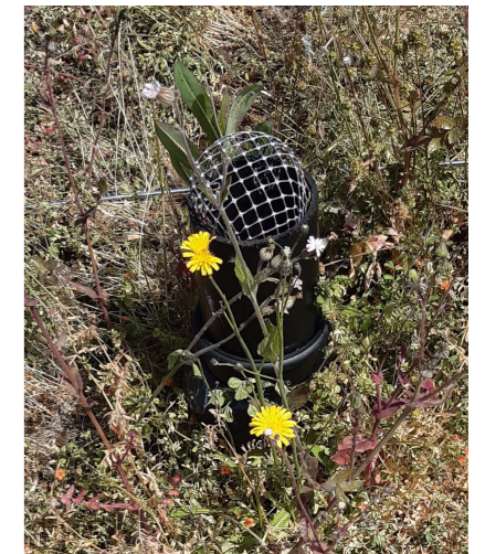
Figure 4. 'Beauty and the Beast!' Wildflowers around a 'stink pipe' on an extensive biodiverse roof.
