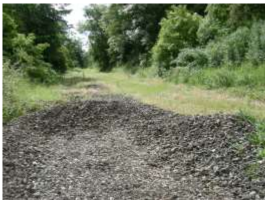
Ballast removal Thornielaw
