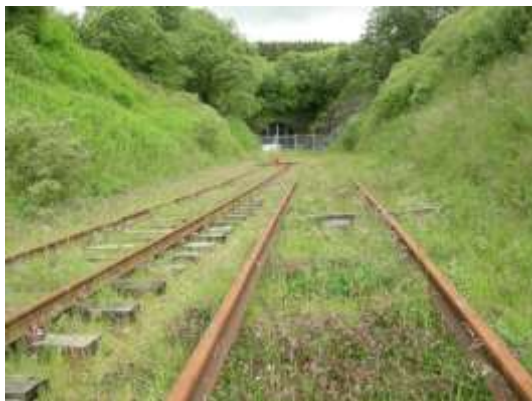
Whitrope Tunnel south entrance 2015
