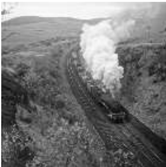
Whitrope Tunnel north entrance
