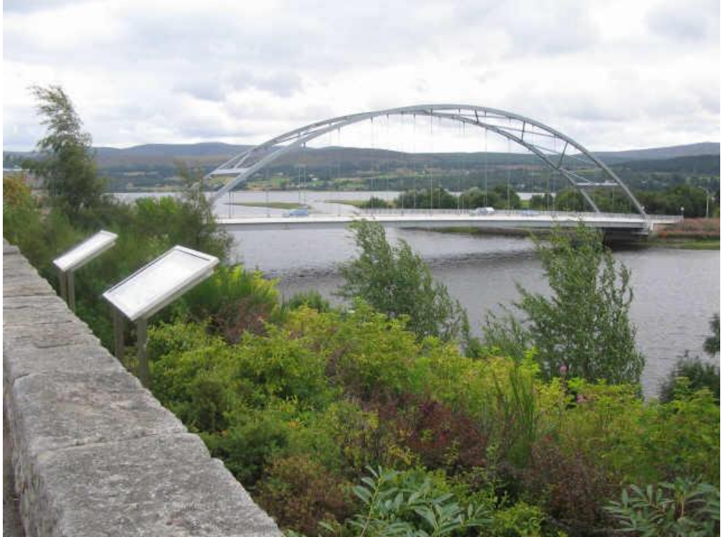
Bonar Bridge from the vc. 107 side looking across the Kyle into vc. 106. Phil Williams.
