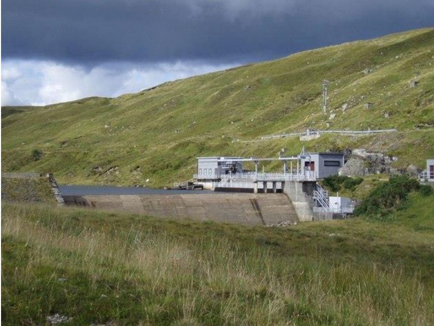
The dam on the R Cassley at Duchally power station NC 36 20. Graeme Smith.
