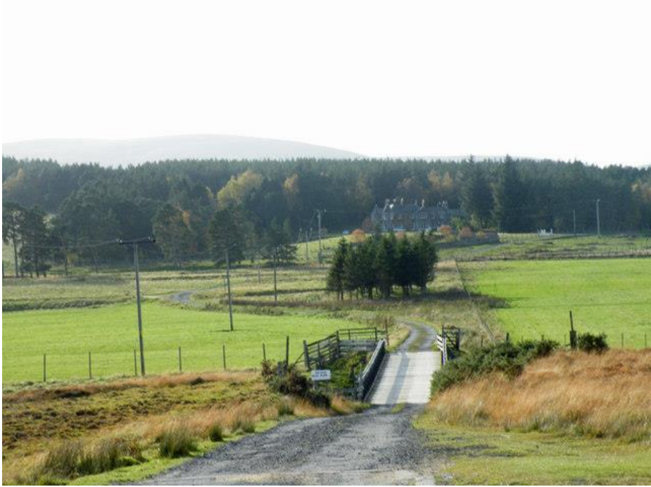
The private road and bridge to Borrobol Lodge. Sarah McGuire.
