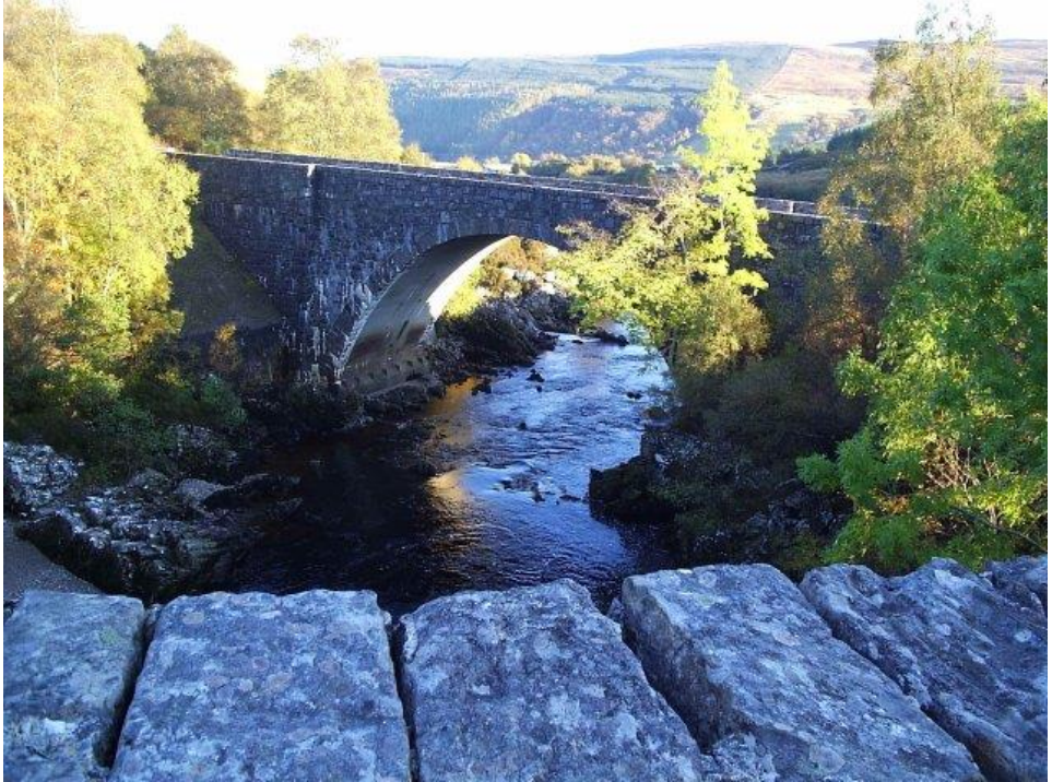
Oykel Bridge from the old road bridge, looking over to the new road bridge. From here downstream, the road is in vc. 107, above the left bank. Donald Bain.
