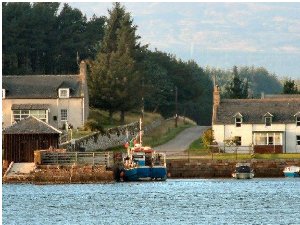
Littleferry Pier from the southern shore of Loch Fleet. Bob Jones.
