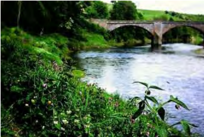
River Tweed at Ladykirk Bridge 1993
