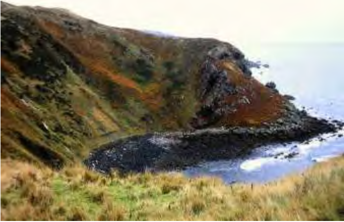
Hilton Bay with new anti-erosion measures 1999
